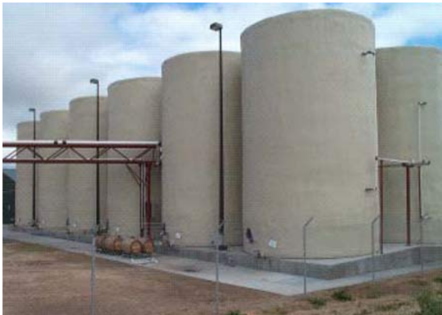
Hand detailing to the tops give the tanks strong crisp visually appealing lines.
